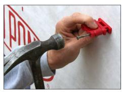
Nail ALINE-SETs to opposite ends of project to be straightened using one or two nails.
